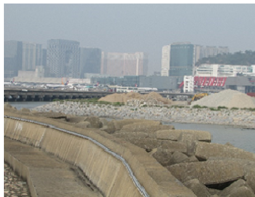
Illustration 14 Data and Power Conduit on Seawall (indicative only)
